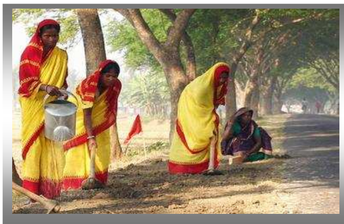
Pic. 1: Female Workers in RIIP Construction Works
